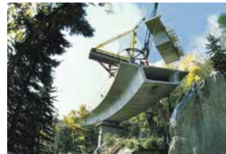
Precast, progressive placement method. Photo Courtesy of Hugh Morton.
