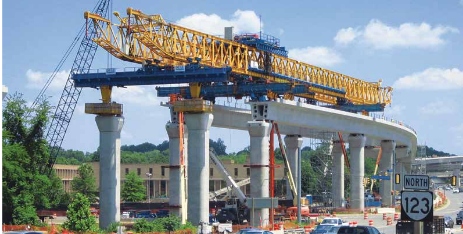
Span-by-span method. Photo Courtesy of Corven Engineering Group, Inc.
