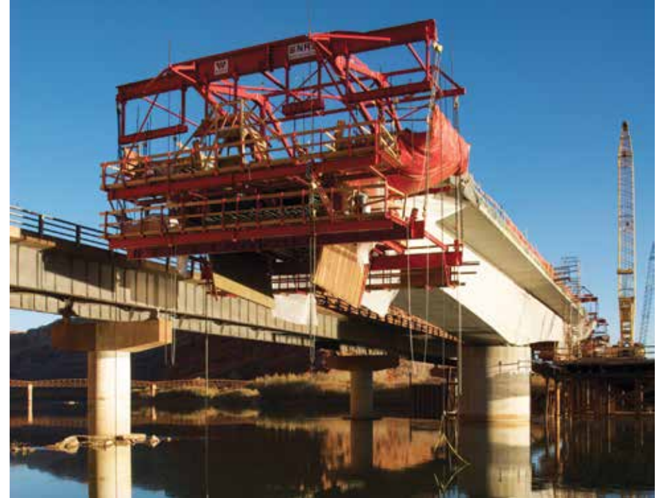
Cast-in-place, balanced cantilever method. Photo Courtesy of FIGG.
