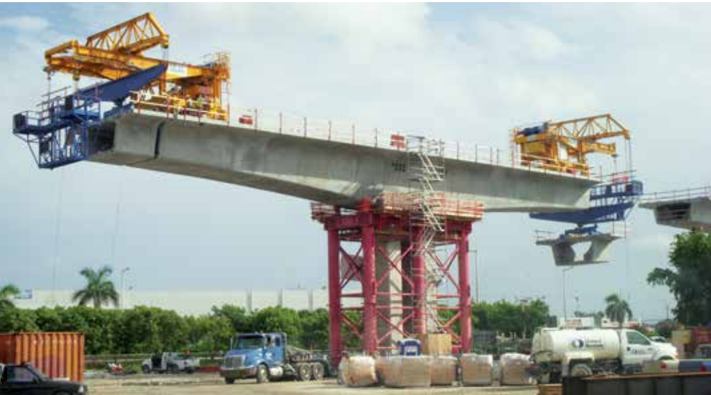
Precast, balanced cantilever method. Photo Courtesy of URS Corporation.
