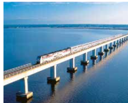
Railway Bridge. Photo Courtesy of AMTRAK, Jim Loomis.
