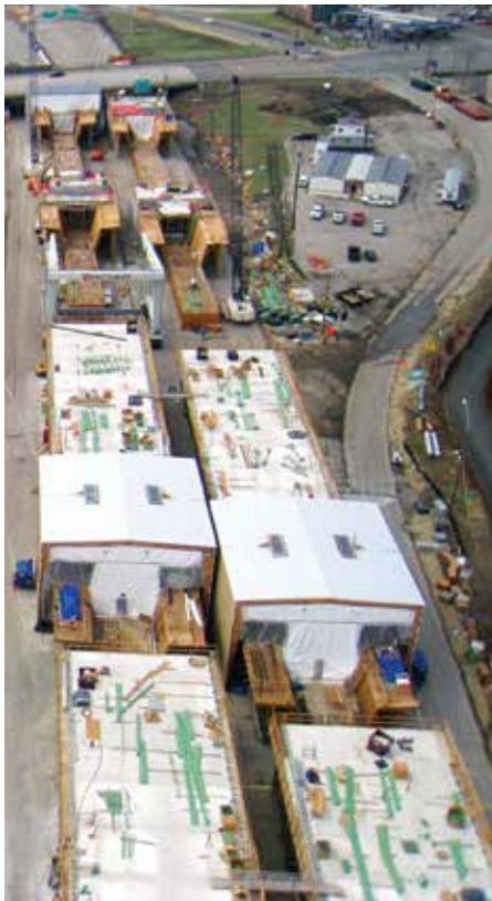
Long-line casting. Photo Courtesy of FIGG.
