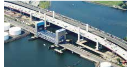
Extradosed bridge. Photo Courtesy of Shoreline Aerial Photography.
