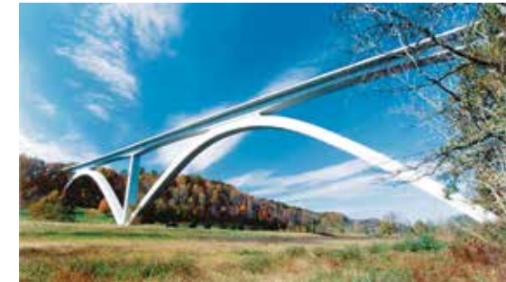
Segmental arch bridge. Photo Courtesy of FIGG.
