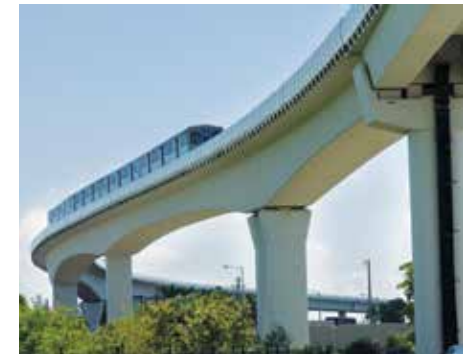
Transit Bridge. Photo Courtesy of URS Corporation.
