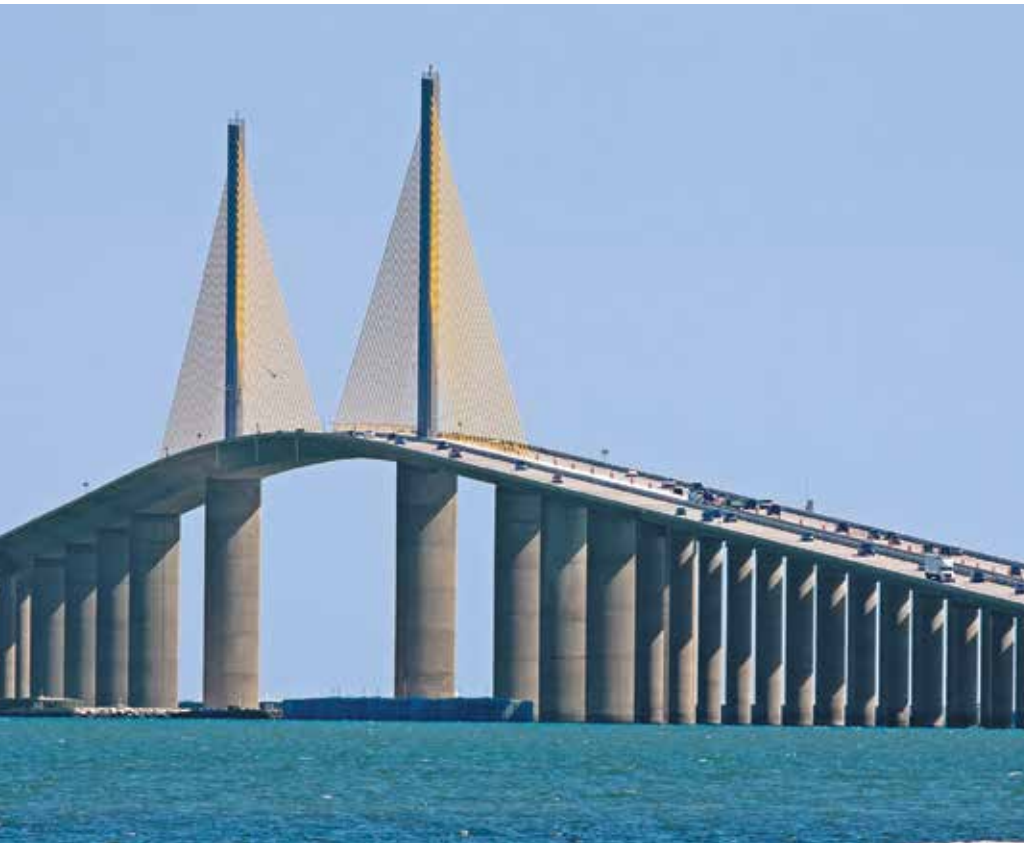
Cable-stayed bridge. Photo Courtesy of Shutterstock.
