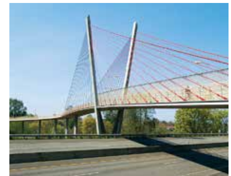
Pedestrian Bridge. Photo Courtesy of OBEC Consulting Engineers.
