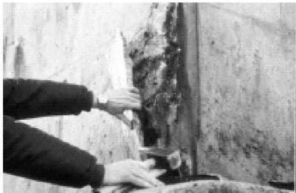
**Figure 9:** Bridge piers exposed to a temperate Nordic marine environment. Extensive damage in the splash zone after 18 years due to chloride induced reinforcement corrosion.
