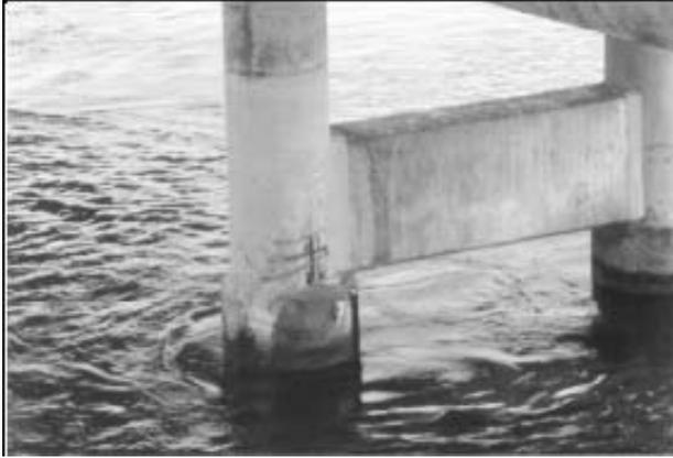
**Figure 29:** Bridge on the Florida Keys. Critical corrosion of epoxy coated reinforcement
