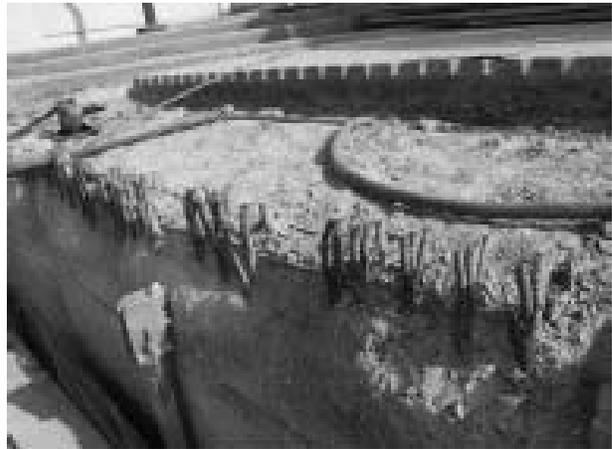
**Figure 31:** Seawall reinforced with epoxy coated reinforcement-heavily damaged by reinforcement corrosion after about 12 years
