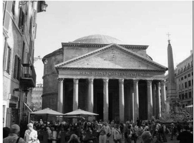
**Figure 3:** Pantheon, Rome. The spherical dome is a 2000 years old concrete structure in full service today.
