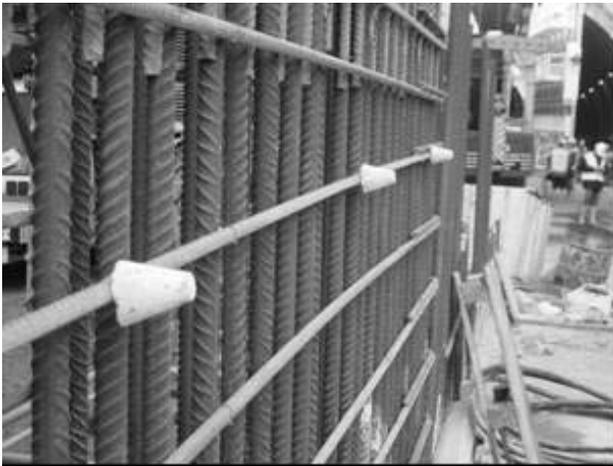
**Figure 37:** Small concrete spacers with large spacing of spacers. Such spacers are not adequate to ensure a reliable concrete cover, as shown on
