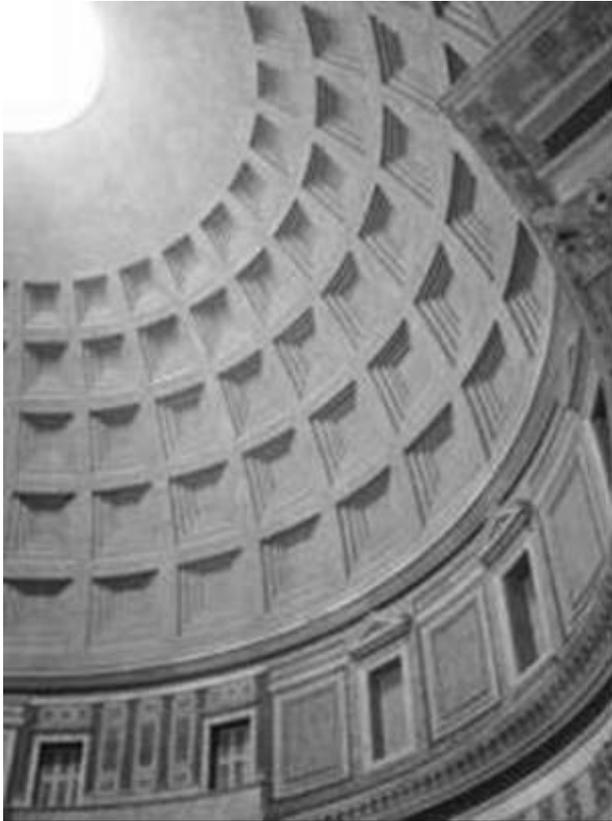
**Figure 42:** The inside of the 2000 years old concrete dome of the Pantheon in Rome shown in Figure 3.
