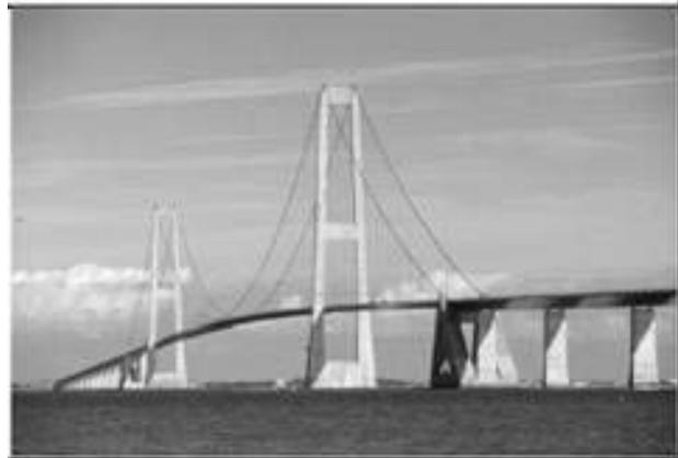
**Figure 13:** Great Belt Link, East Bridge. Denmark. Central span L=1416m. Design Life: 100 years.
