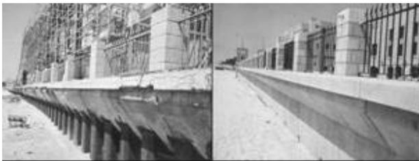
**Figure 43:** A reinforced concrete capping beam on top of a steel sheet pile seawall. To the left, the extensive reinforcement corrosion after 4-5 years requiring replacement of the capping beam. To the right the new capping beam, but now made from unreinforced concrete. This new structure has now served problem-free for more than 15 years.
