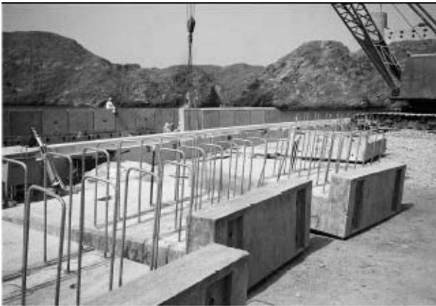
**Figure 27:** Stainless steel reinforcement used in the precast structural members to replace a corrosion damaged seawall protecting the existing important buildings and the new Building Complex (Figure 26) from the Gulf.
