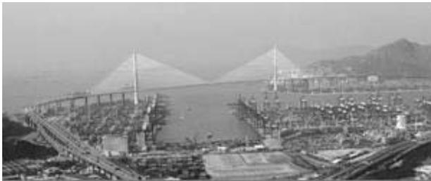
**Figure 24:** Stonecutters Bridge, Hong Kong. The outer layer of reinforcement in the pylons is Stainless steel reinforcement; the remaining reinforcement is ordinary black steel reinforcement. Construction has just started. Design: COWI A/S in Joint Venture with Arup. (Model photo).
