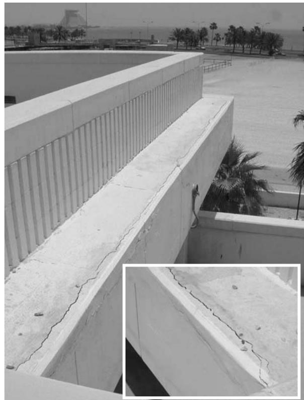
**Figure 5:** With moisture and aggressive substance penetrating the surface as illustrated in Figure 4, it becomes evident that edges are exposed from more than one side, thus leading to concentration of the nasties and early deterioration starting at the corners - the so-called "corner effect".
