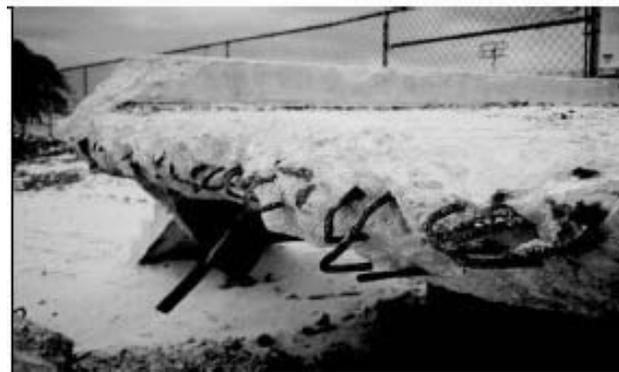
**Figure 12:** Close-up of the land based remaining parts of the “new” pier of which part of the remaining piles are shown in Figure 11. This pier was reinforced with ordinary black steel reinforcement and lasted only about 10 years.
