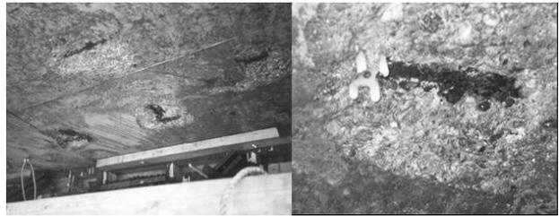
**Figure 40:** A systematic set of spalled concrete is clearly visible of the underside of the box girder of Figure 39, as seen to the left. The reason is documented on the close-up to the right: The use of plastic spacers. Plastic spacers are not compatible with concrete and should not be used in highly corrosive environments.
