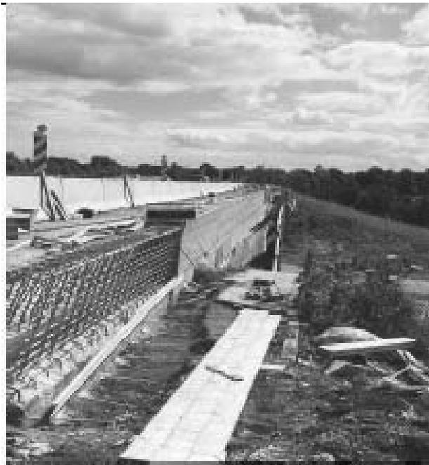
**Figure 28:** Replacing edge beams and parapets on Danish bridges and crash barriers on the motorways exposed to de-icing salt. SSR is introduced to avoid future repairs as well as avoiding the serious delays and inconveniences to the users, an issue becoming more and more in focus with the growing awareness of the costly societal consequences of such delays.
