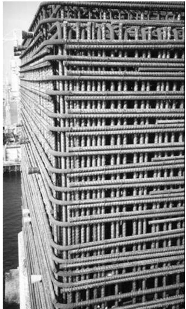
**Figure 34:** Example of reinforcement detailing which does not respect the need for reliable casting and compaction of concrete. Particularly the quality of the concrete cover, the "skin", is in danger
