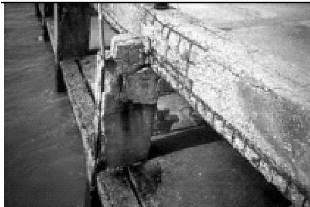
**Figure 8:** Reinforced concrete jetty in the Gulf exhibiting extensive chloride induced corrosion damage with delamination already after 2-3 years, and having reached a stage of failure and collapse after 7.5 years when this picture was taken.
