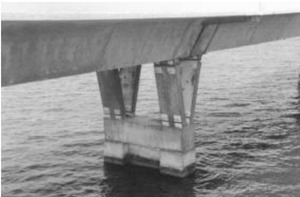
**Figure 30:** Bridge on the Florida Keys. Critical corrosion of epoxy coated reinforcement leading to splitting of the V formed supports now strengthened by prestressed bolts
