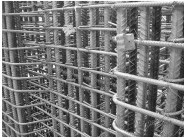
**Figure 25:** Illustration of the selective adoption of SSR in the outer layer of reinforcement in a highly corrosive environment. The reinforcement layers behind are ordinary black steel reinforcement.
