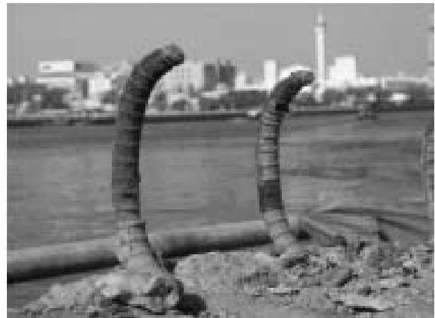
**Figure 32:** Close-up of the corroded epoxy coated reinforcement shown on Figure 31.
