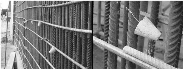
**Figure 38:** The small concrete spacers shown on Figure 37 have no stability and cannot be fixed adequately. In view of the importance of achieving the correct concrete cover, this situation is not acceptable.
