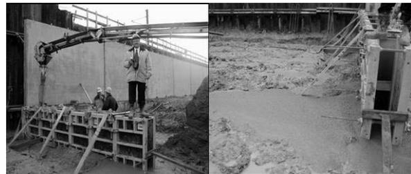
**Figure 36:** Self Compacting Concrete, SCC. Left: uniformly filling the form by pouring the concrete into one end of the form. Suddenly the concrete stopped rising in the form. Right: The reason being that a small slot in the form let the SCC flow out of the form! Conclusion: Formwork for SCC shall be (water-) tight, and also stronger than usual to resist the increased form pressure.
