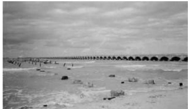
**Figure 11:** 65 year old stainless steel reinforced pier at Progreso in Mexico still fully intact without maintenance whereas the remains in the foreground is what is left of an only about 30 year old pier reinforced with ordinary black steel reinforcement, see Figure12, [17].
