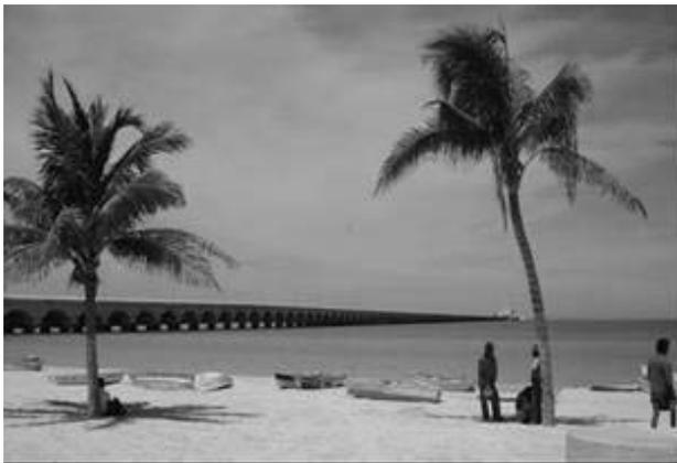
**Figure 10:** The 2.2 km long pier into the Gulf of Mexico at Progreso, built 65 years ago and in full operation today carrying heavy container lorries back and forth from a new container terminal built further out at sea. The piers are reinforced with stainless steel reinforcement as described in [1].
