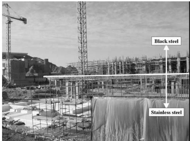
**Figure 26:** Overview of the construction site of a seaside Building Complex. Stainless steel
