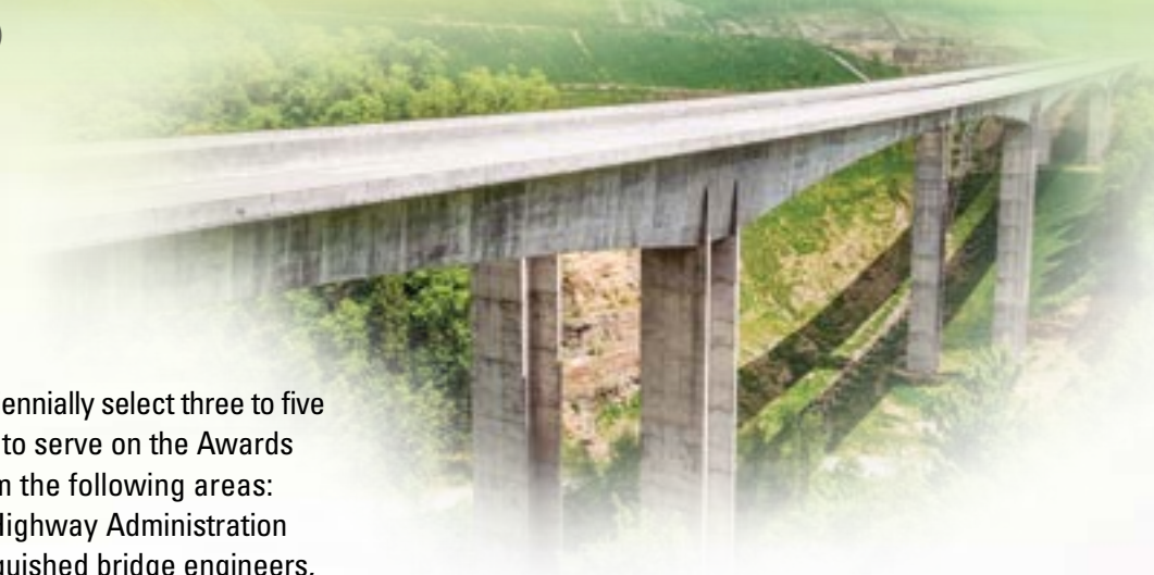
Route 460 Connector Phase I – Grassy Creek Bridges Owner: Virginia Department of Transportation – Bristol District Photo Courtesy of Jason Schneider
