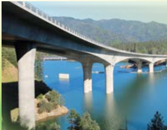
I-5 Antlers Bridge Replacement Owner: Caltrans Photo Courtesy of Caltrans
